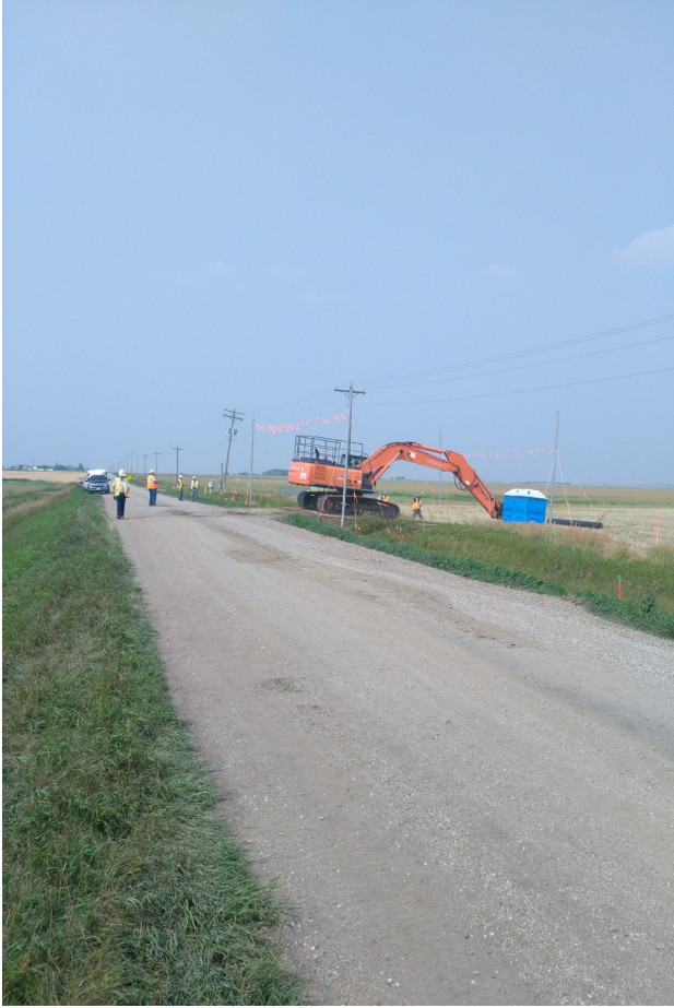
Access to ROW at road 59 Black Creek
